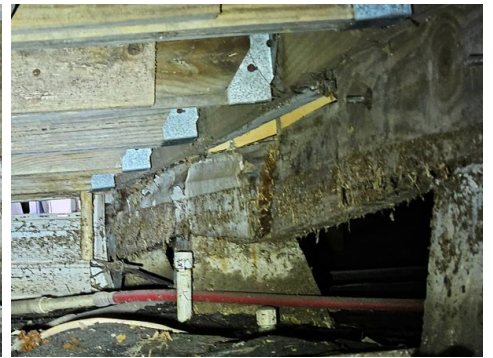
Damaged Floor Joist
