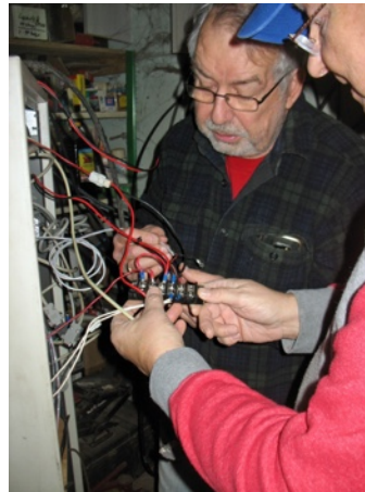
Jim, W2JTC working on the DC power distribution with Gary
