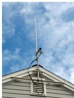
Aluminum angle irons hold a mast above my garage. On top of the mast is a VHF/UHF vertical antenna. Mounted on a short standoff is a dipole antenna fed with window line going to a AH-4 remote tuner just inside the garage wall.
