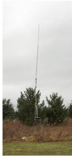
Living on 12 acres they have plenty of room for antennas. For the HF bands there is a full size 160 meter balanced dipole system fed with twin-lead operating on all bands. Also there is a ground mounted trap vertical and an elevated 20 meter vertical with eight radials. The elevated vertical is his primary DX antenna. You will also find a 6 meter ground plane and a VHF/UHF vertical. All antennas are homemade except the VHF/UHF vertical.
