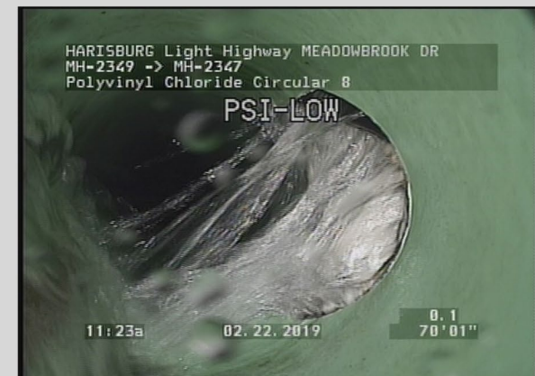
Leaking Sewer Lateral Connection
