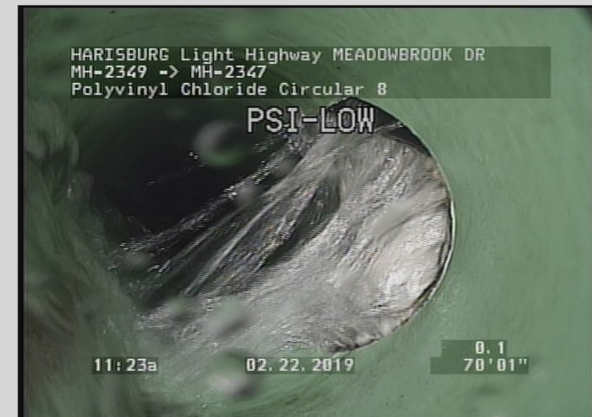
Leaking Sewer Lateral Connection
