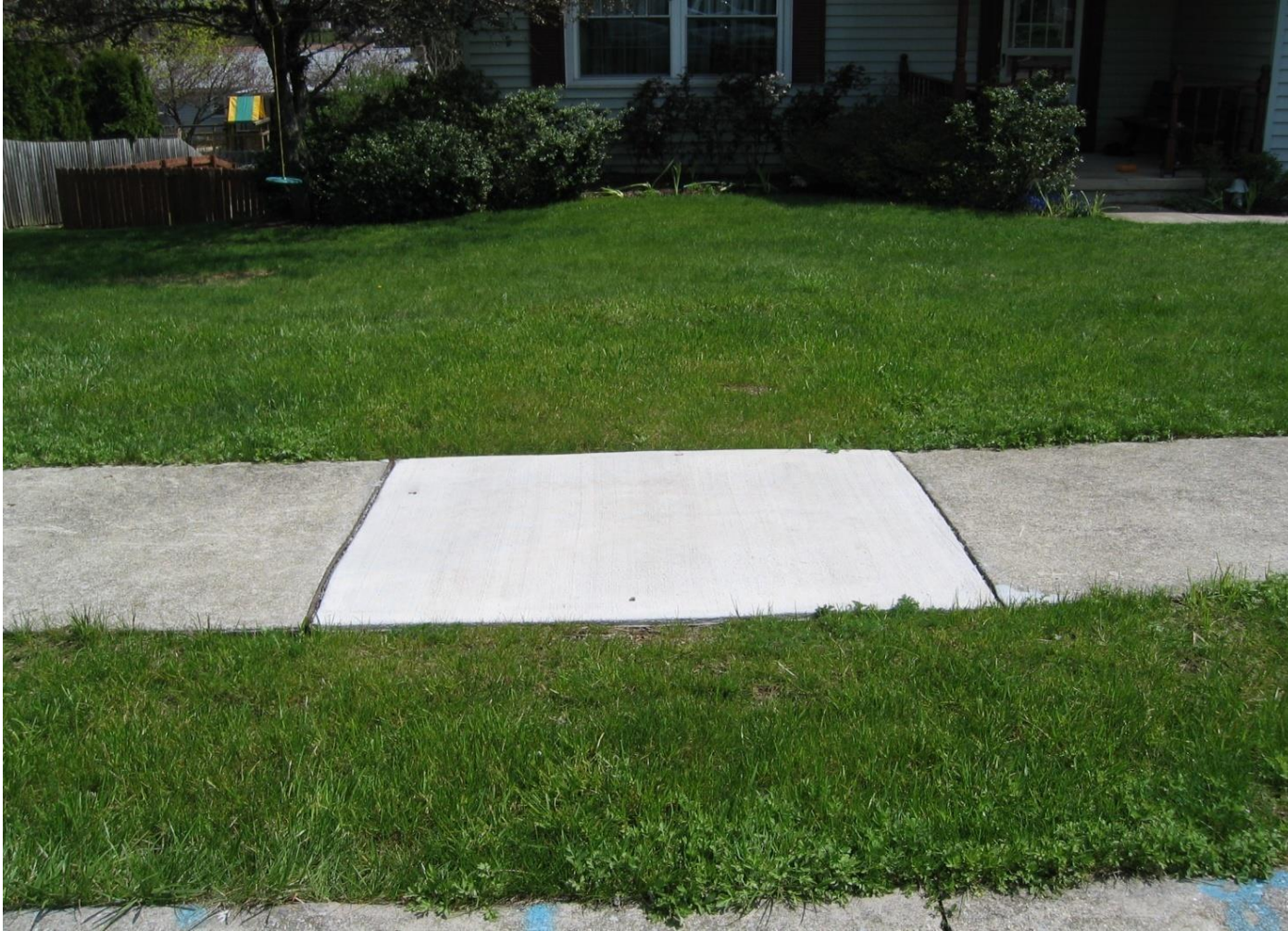
Typical Sidewalk and Lawn Restoration
