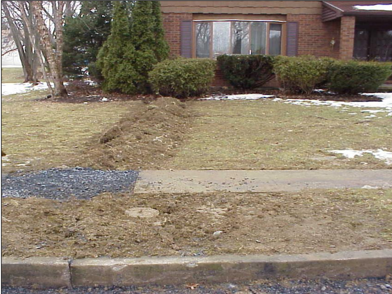
Typical building sewer replacement (prior to restoration)
