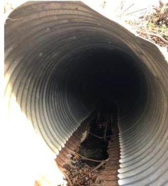
The project will replace the failing infrastructure with new modern materials such as smooth lined corrugated polyethylene pipe and PennDOT standard pre-cast concrete drainage structures.
