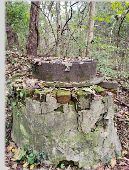
Deteriorated Brick Manhole in SC-2B
