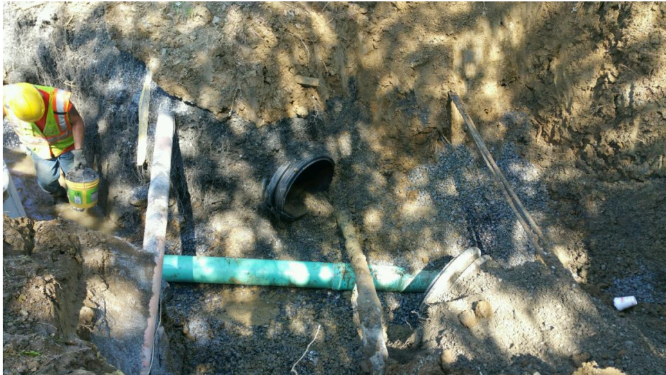
Once buried, it is difficult to identify issues with underground utilities
