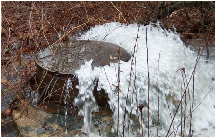
Photo showing sanitary sewer overflow out of a manhole
