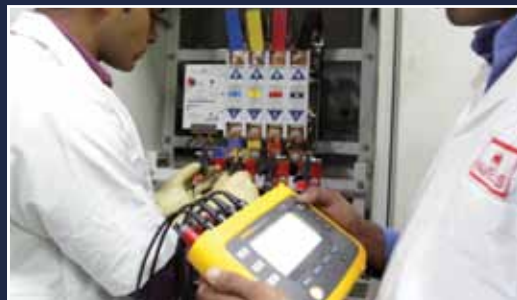
LOAD FLOW & HARMONICS ANALYSIS
