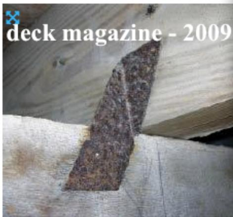
**Figure 1. Many new wood treatment chemicals are more corrosive than the old CCA. Hardware that once could be depended on to last for decades now may degrade in only a few years.**
