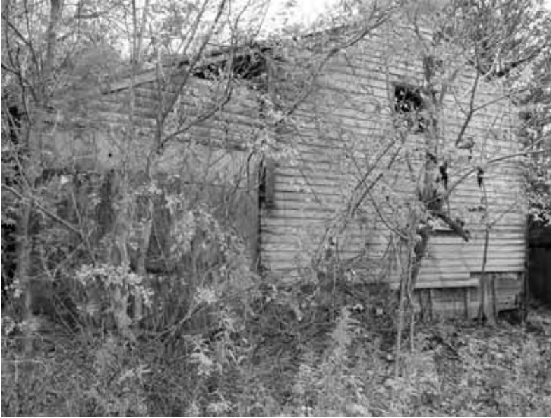
Figure 1 CP198_02. View to the southwest.
