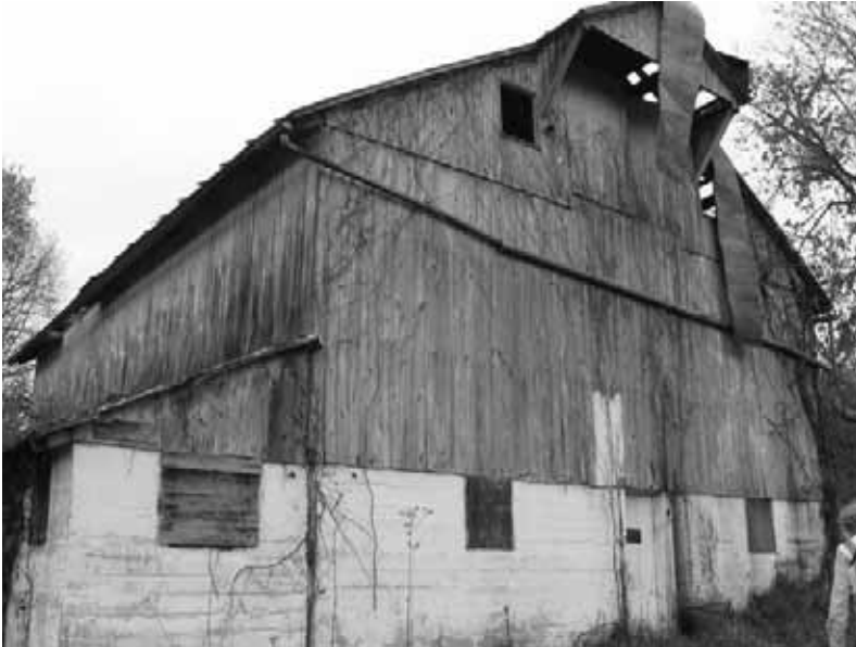
Figure 3 CP197_04. View to the southwest.
