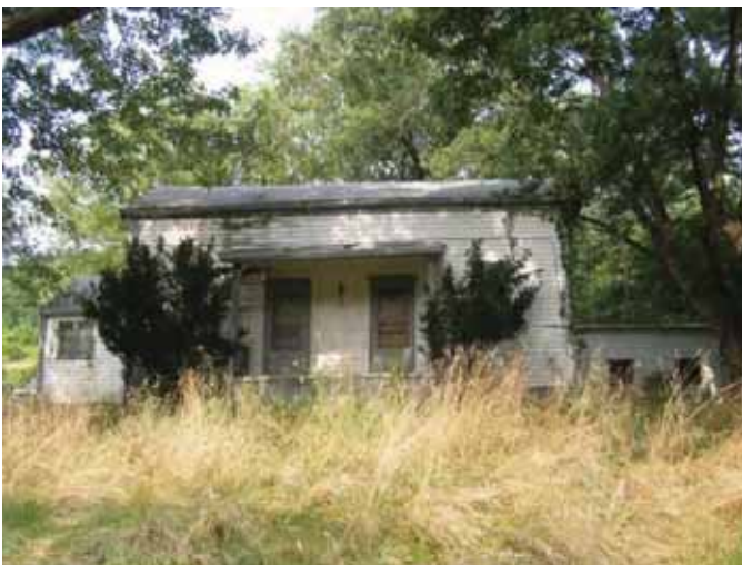
Photograph 5 Tratt House, view west
