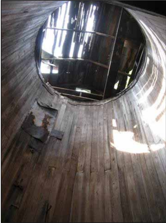
Silo Interior, July 28, 2009
