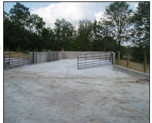
Animal waste handling system - one of the approved Best Management Practices through the Soil Erosion and Water Quality Cost Share Fund.
