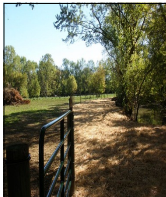
Animal trail and walkway installed on a horse farm through the Alternative Agriculture Grant.
