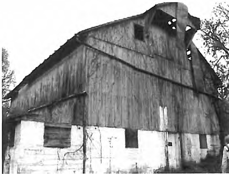
Figure 3 CP197_04. View to the southwest.
