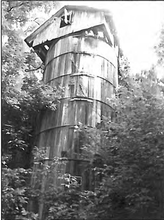
Wood Silo, July 28, 2009
