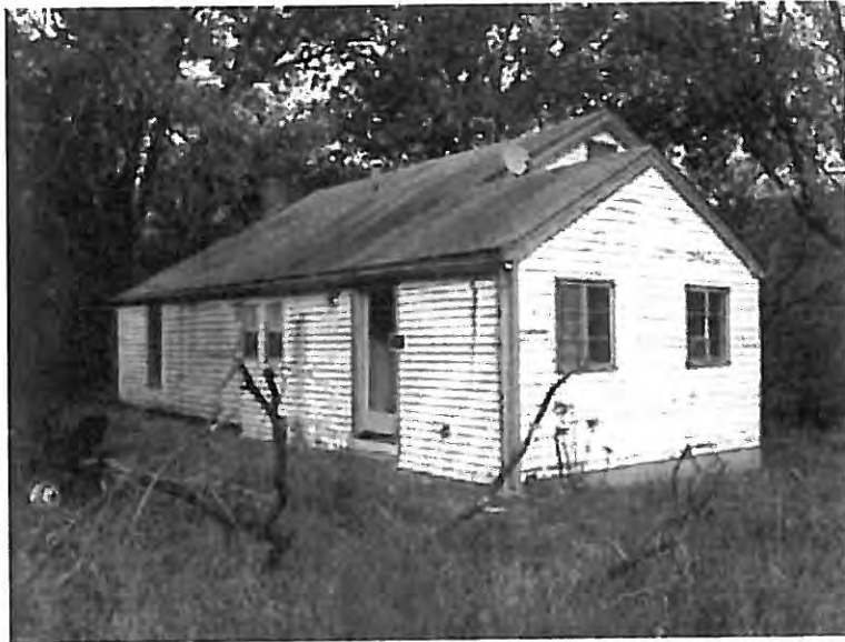
Figure 2 CP197_03. View to the southeast.
