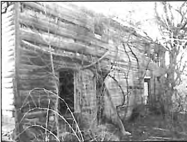
Photograph 4 Ware House, view southeast
