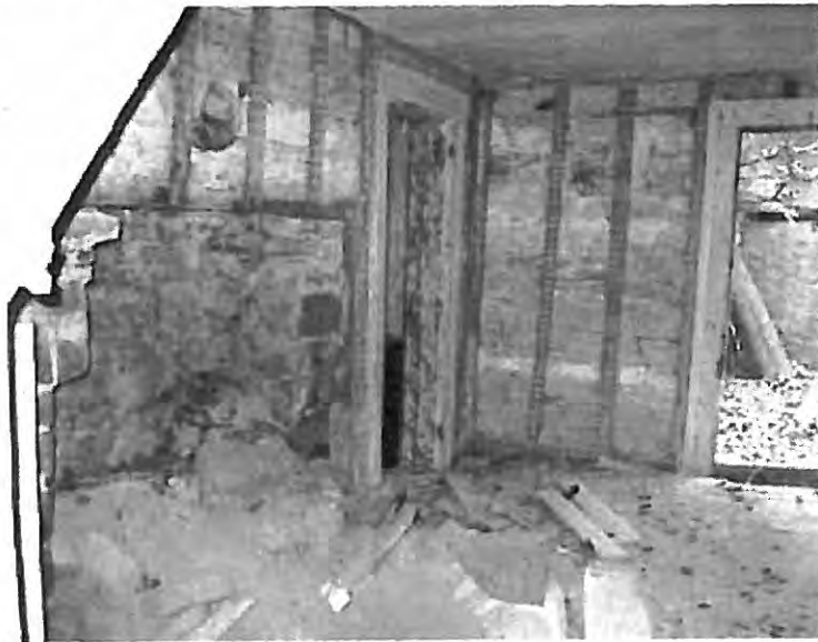
Figure 2 CP198_03. View to the west.
