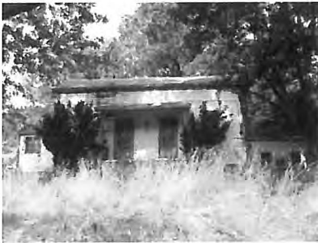
Photograph 5 Tratt House, view west
