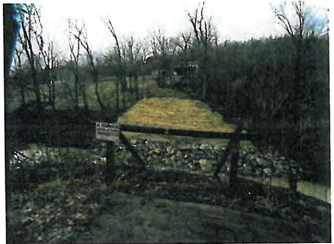
Bridge area after removal of bridge - looking west.
