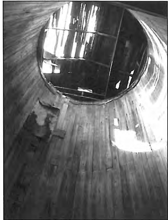
Silo Interior, July 28, 2009
