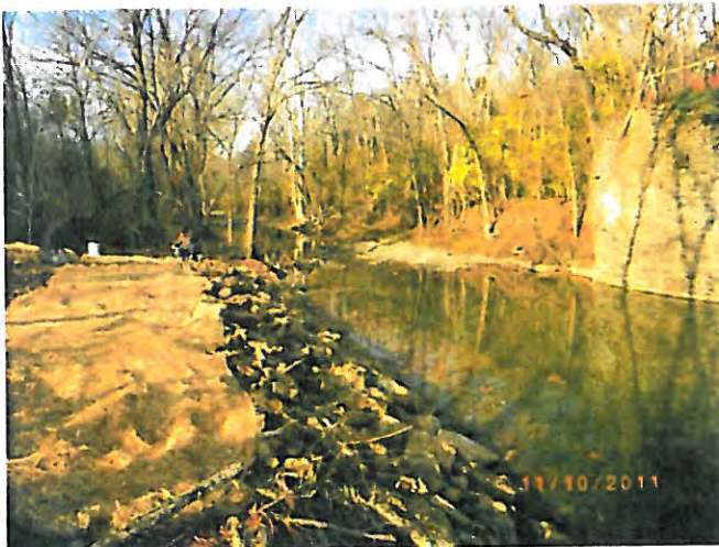
Bridge area after removal of bridge - looking north.
