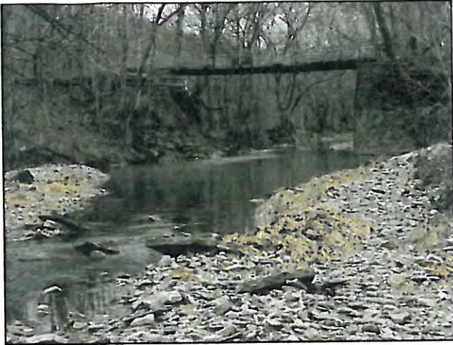
Trailer frame bridge across Riffle Creek
