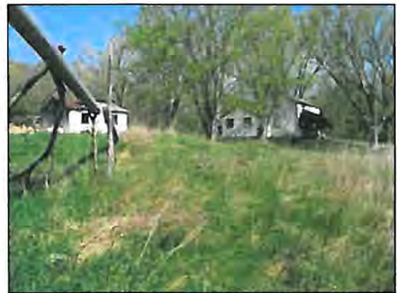
House and Outbuilding in Area B - Overgrown Lawn and Pasture
