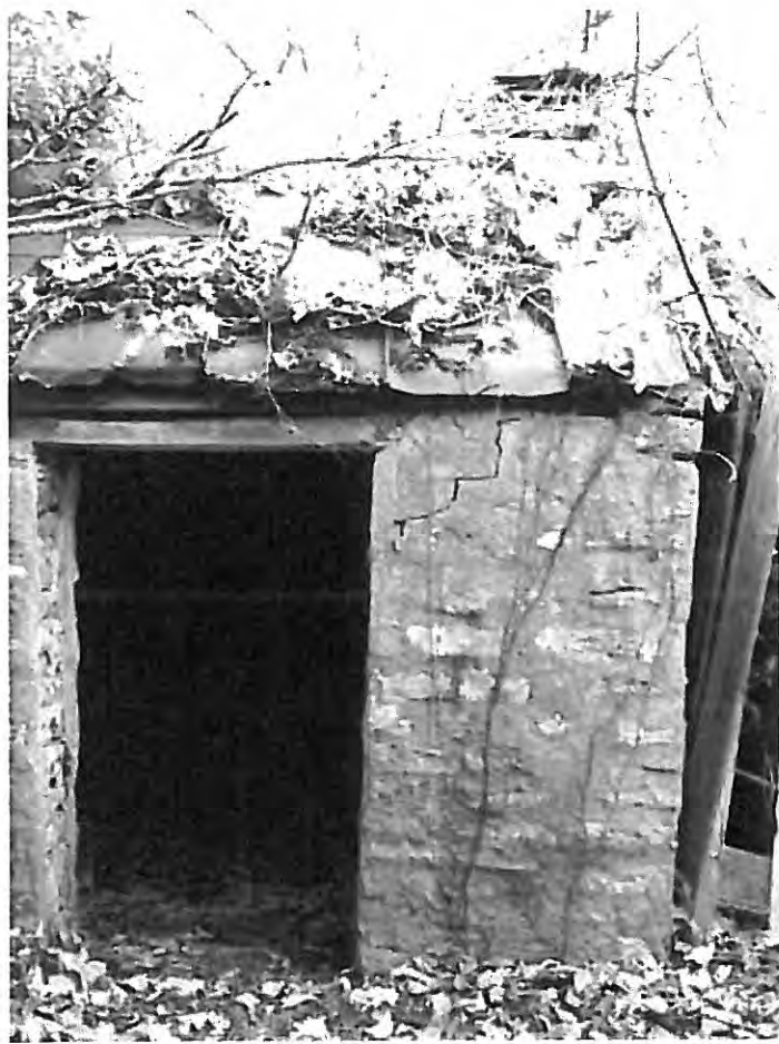
Figure 3 CP198_04. View to the west.
