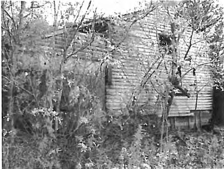
Figure 1 CP198_02. View to the southwest.
