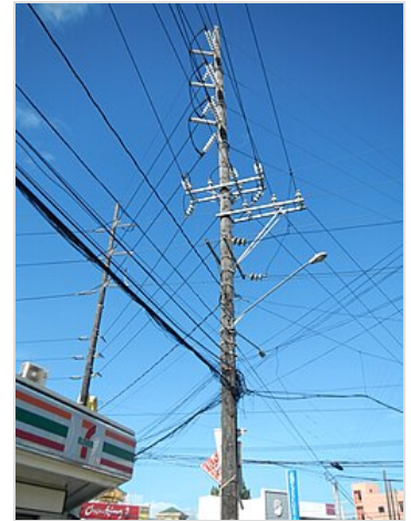
A 115 kV subtransmission line in the Philippines , along with 20 kV distribution lines and a street light , all mounted on a wood subtransmission pole
