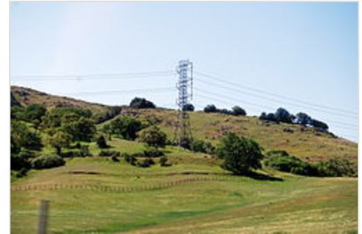
A high-power electrical transmission tower, 230 kV, double-circuit, also double-bundled
