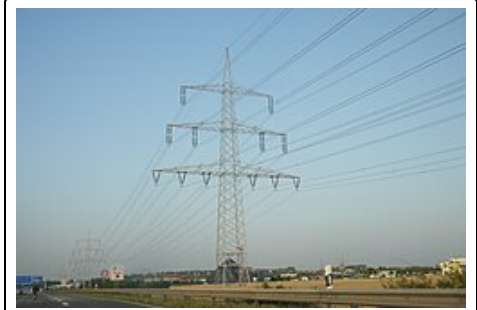
A four-circuit, two-voltage power transmission line; Bundled 2-ways
