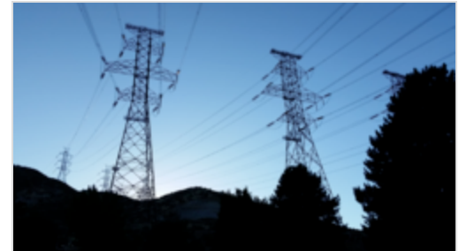
Five-hundred kilovolt (500 kV) Three-phase electric power Transmission Lines at Grand Coulee Dam. Four circuits are shown. Two additional circuits are obscured by trees on the far right. The entire 6809 MW [1] nameplate generation capacity of the dam is accommodated by these six circuits.
