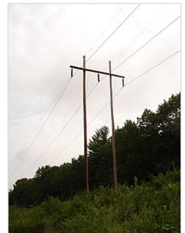
115 kV H-frame transmission tower
