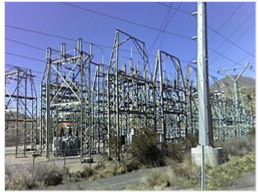
A transmission substation decreases the voltage of incoming electricity, allowing it to connect from long-distance high-voltage transmission, to local lower voltage distribution. It also reroutes power to other transmission lines that serve local markets. This is the PacifiCorp Hale Substation, Orem, Utah, US .
