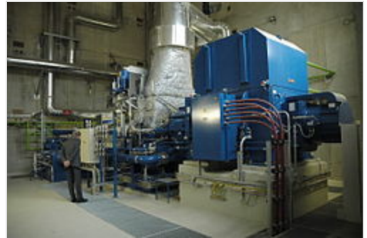
A direct-drive 5 MW steam turbine
