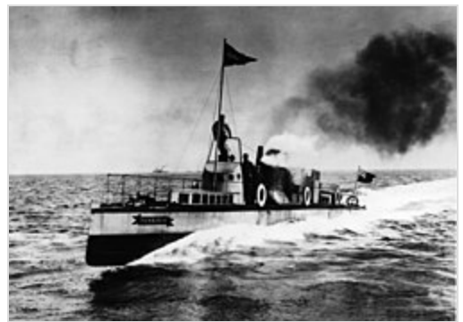
Turbinia , 1894, the first steam turbine-powered ship
