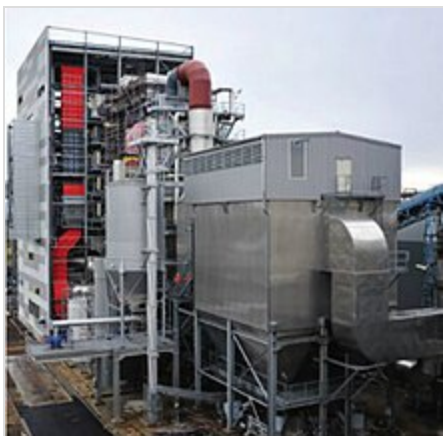
A cogeneration plant in Metz, France. The 45 MW boiler uses waste wood biomass as an energy source, providing electricity and heat for 30,000 dwellings.
