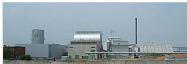
Masnedø CHP power station in Denmark . This station burns straw as fuel. The adjacent greenhouses are heated by district heating from the plant.
