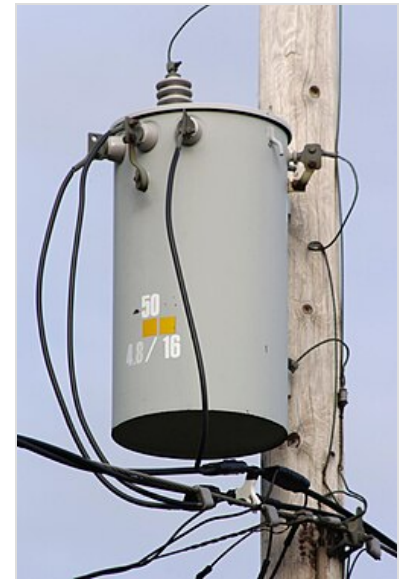
A 50 kVA pole-mounted distribution transformer
