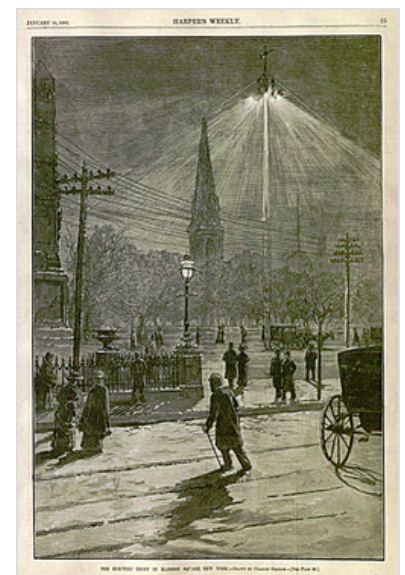
The late 1870s and early 1880s saw the introduction of arc-lamp lighting used outdoors or in large indoor spaces, such as this Brush Electric Company system installed in 1880 in New York City .
