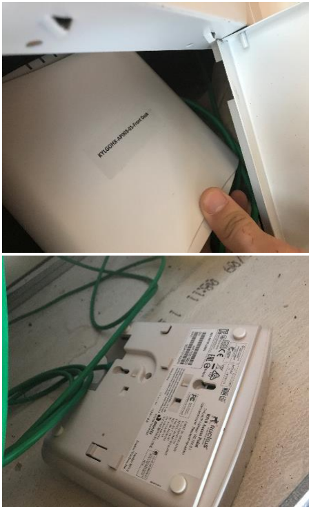
Typical Public R510 in Ceiling Tile or Access Panel
