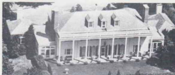
The Asa Bushnell Center — ECAC Headquarters
