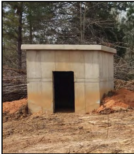
Pre-Cast grenade bunker
