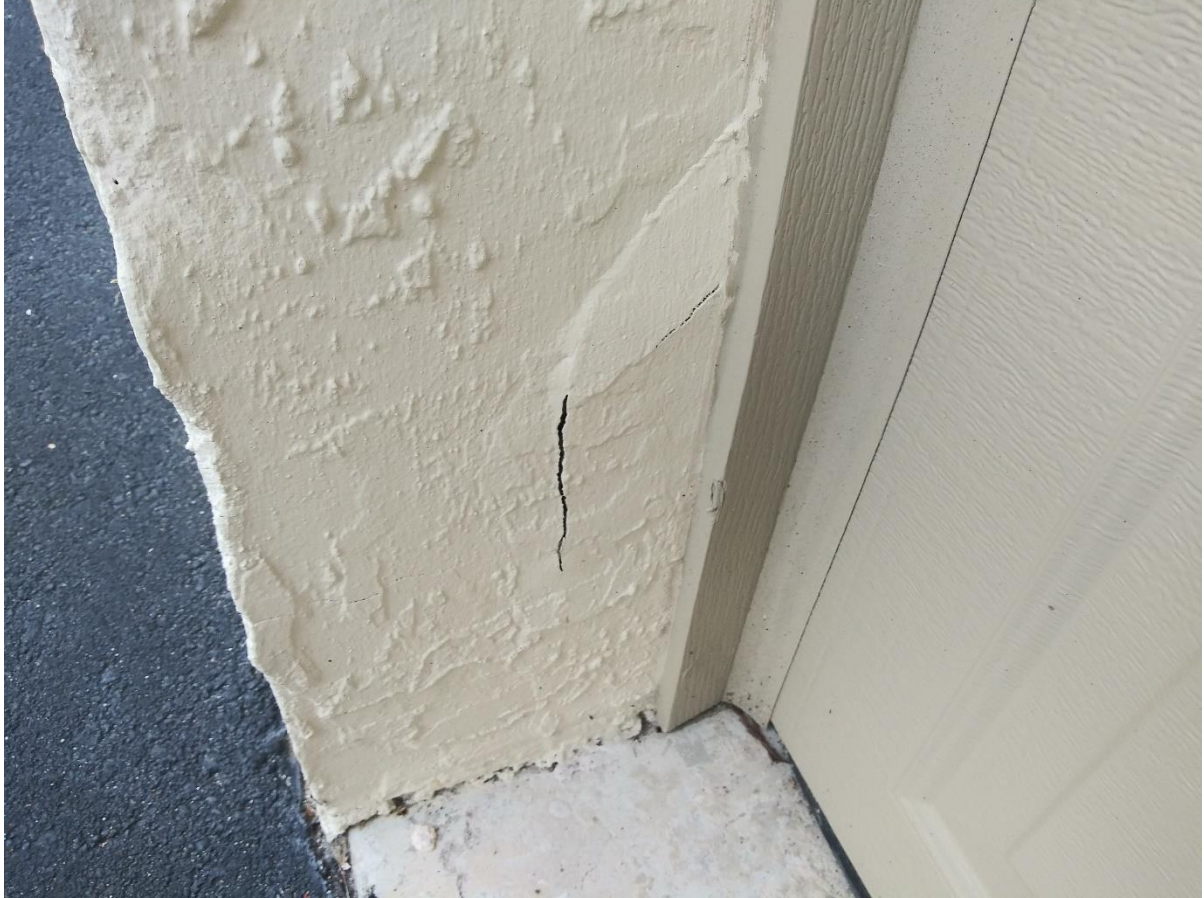
Figure 2: 201 C Garage Crack
