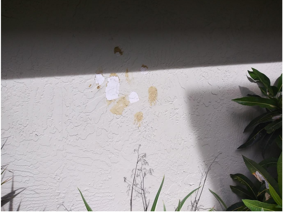
Figure 3: 201 C Garage Paint
