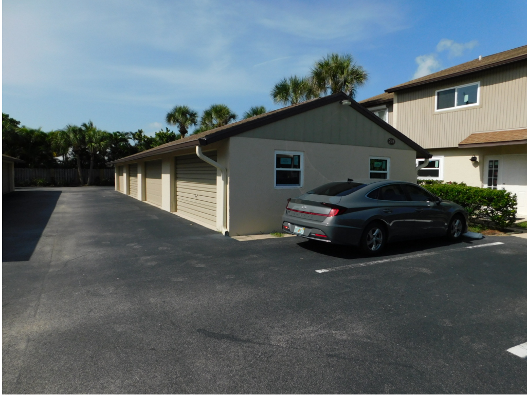
Representative Parking Garage Building Front View
