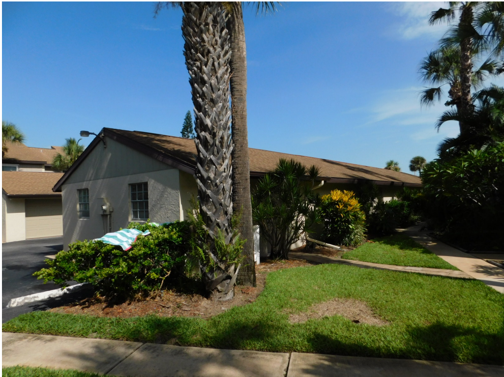
Building Rear View
