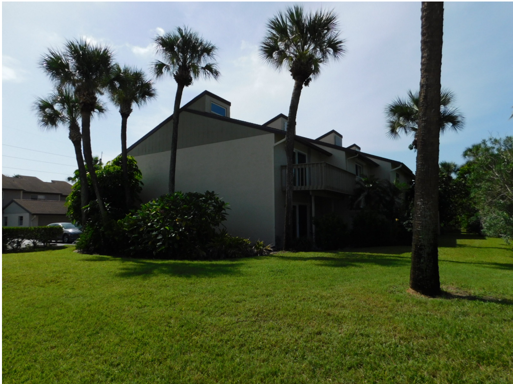
Building Rear View
