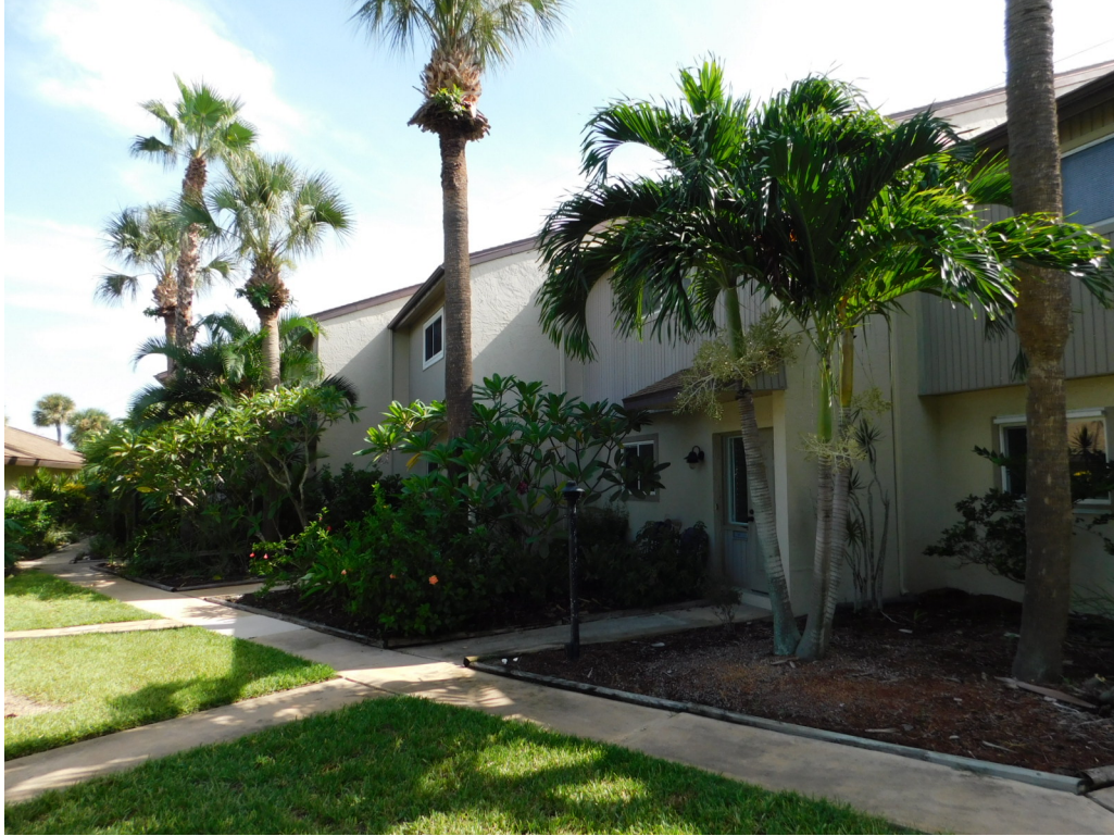
Representative Building Front View
