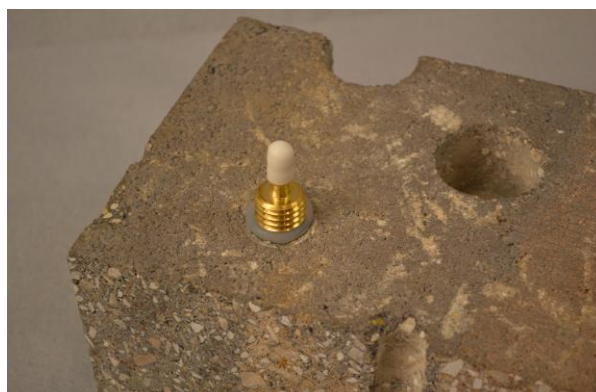
Figure 3. Installed VAPOR PIN®
