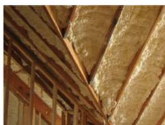
**Keep a Tight Lid on It: Spray Foam Insulation within an Unvented Attic**
