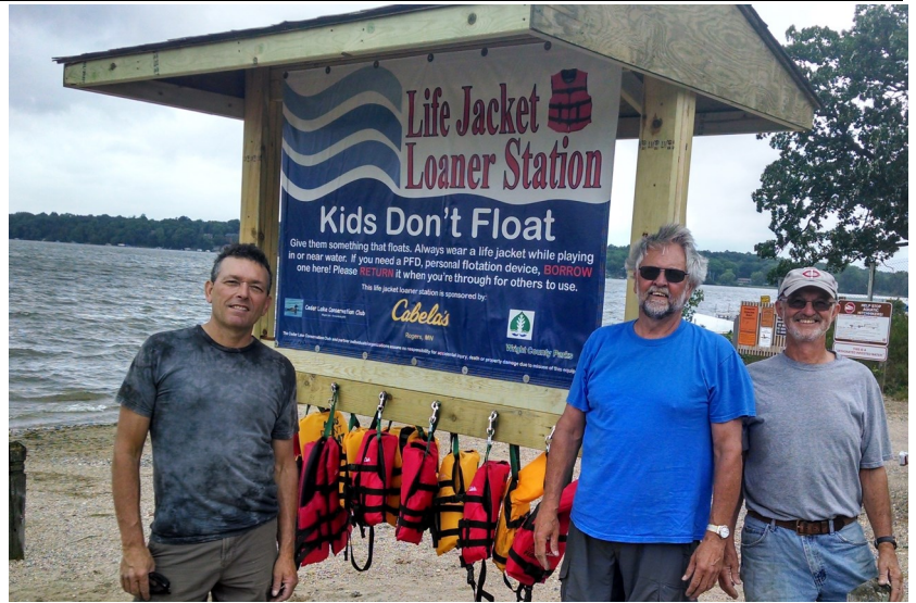
CLCC Members (from the left) Mark Grimme, Glenn Baird, and Dean Nicholson installing the station
