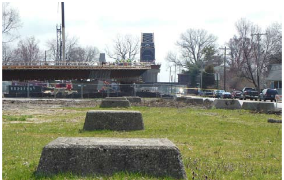
Concrete piers from the Big Four Railroad Bridge line Mulberry Street in Jeffersonville in this March 2013 photo by Charles W. Arrington.
