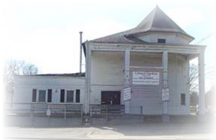
Colonial Gardens on New Cut Road is undergoing restoration and adaptive reuse.
