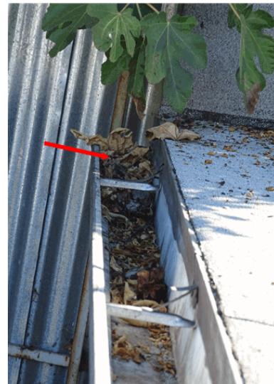
Gutter filled with debris.
