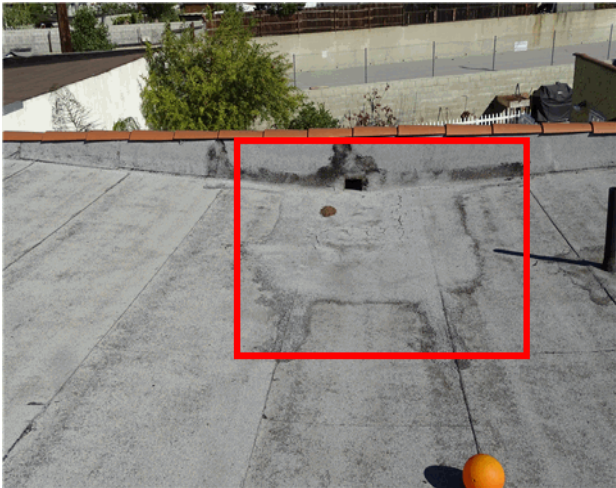
water stain, rolled roof has cracks.
