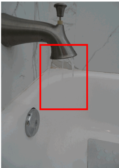
Diverter valve leaking.
