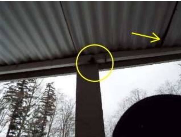
Photo 9-1 Underneath backyard deck
