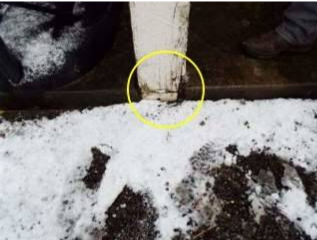
Photo 17-1 South side post under deck
