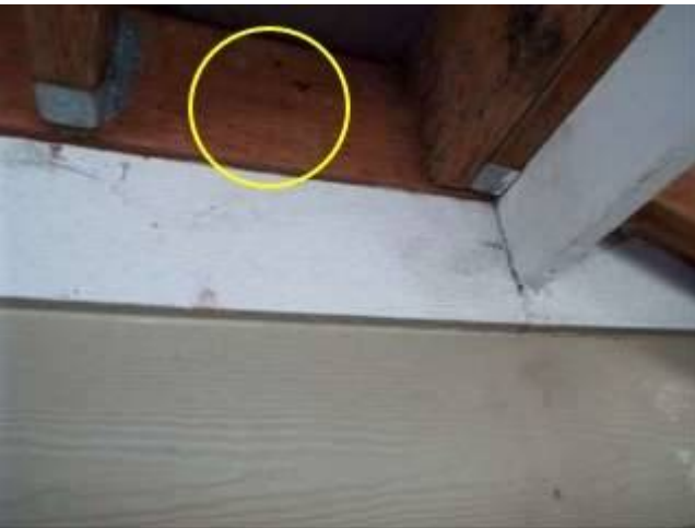
Photo 7-1 Underneath backyard deck
