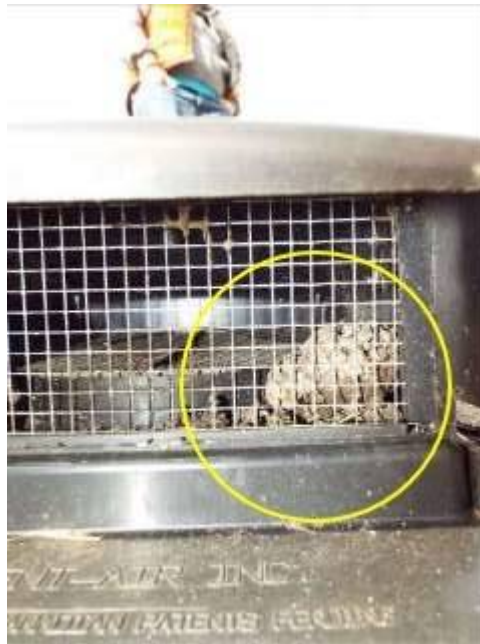
Photo 32-2 South side of roof in vent
