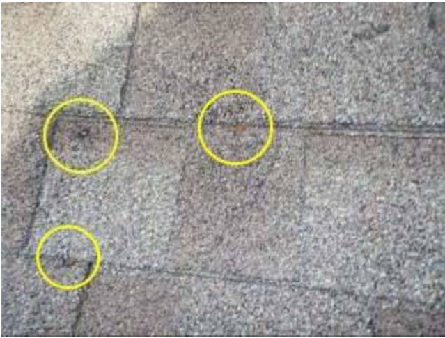
Photo 33-1 South side of roof
