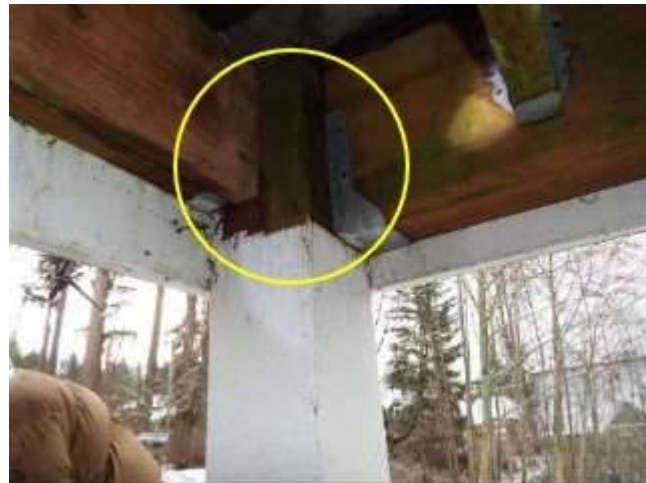
Photo 9-2 Post holding south west corner of deck in backyard
