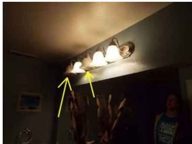
Photo 41-2 Master bath room
