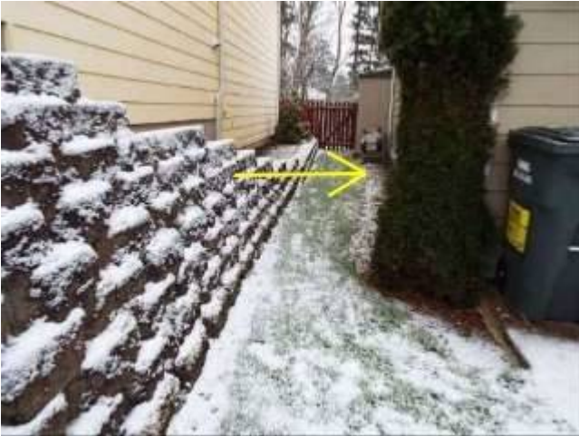
Photo 4-1 East North corner of house
