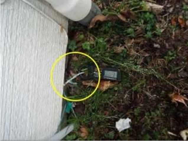
Photo 37-1 East side of house
