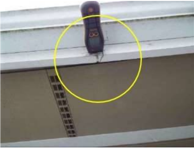
Photo 14-1 On south side of house
