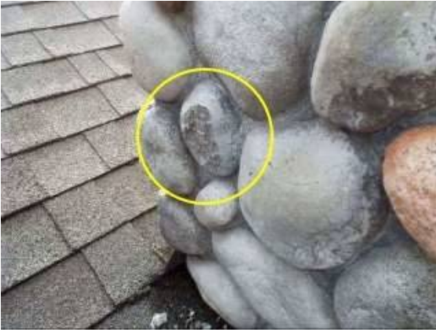
Photo 46-1 East side of chimney
