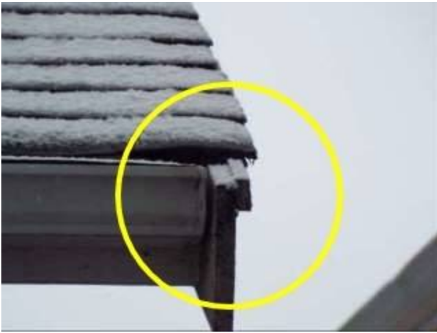
Photo 27-1 South east corner of roof
