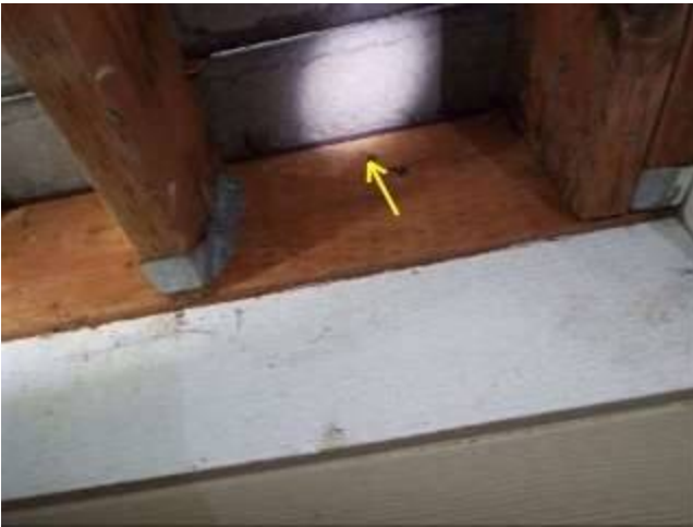
Photo 6-1 Underneath backyard deck
