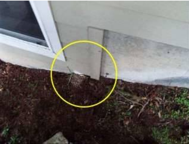
Photo 15-1 South side of house
