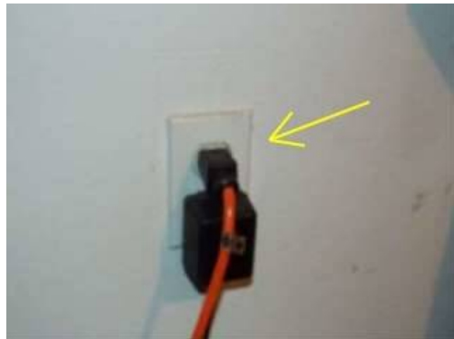
Photo 38-2 South wall of Garage
