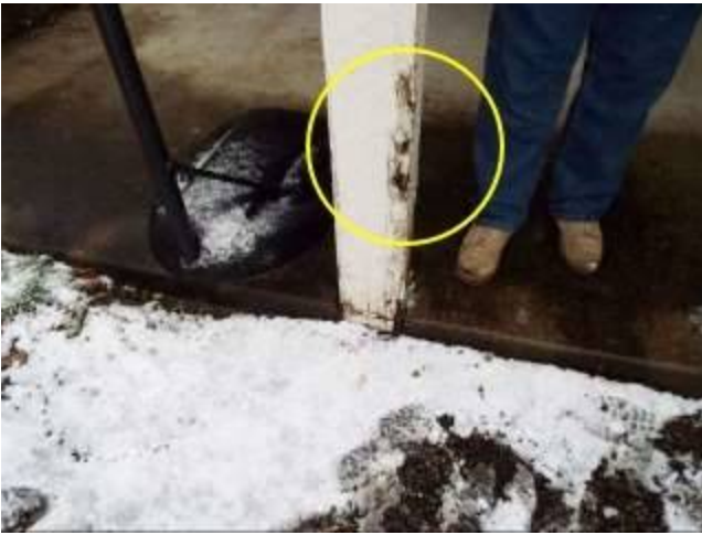
Photo 16-1 Under backyard deck
