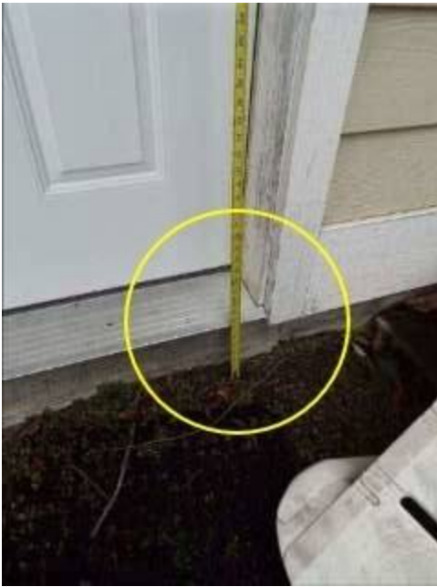
Photo 8-1 Rear garage door that goes into backyard
