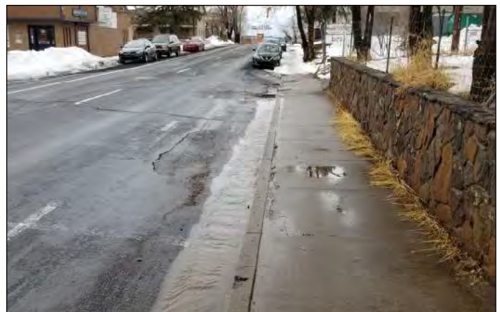
AFTER: Inspector locates and clears blocked inlet.
