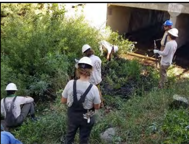
Conservation crew removing vegetation from channel.
