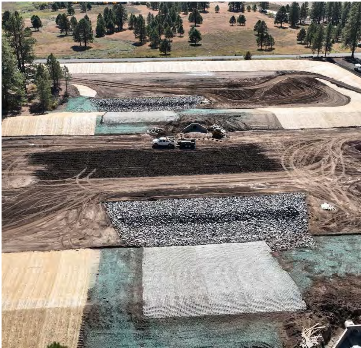
Schultz Creek Flood and Sediment Detention Basin construction.
