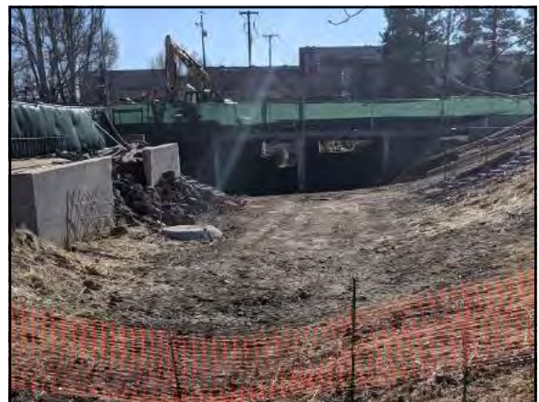
Over-excavation of the ADOT Milton Bridge for future RDF Tunnel.
