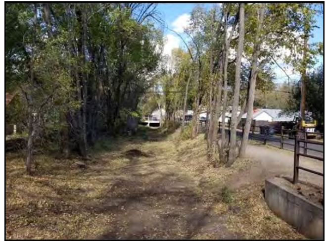
Siberian elm removed from channel and lower banks.
