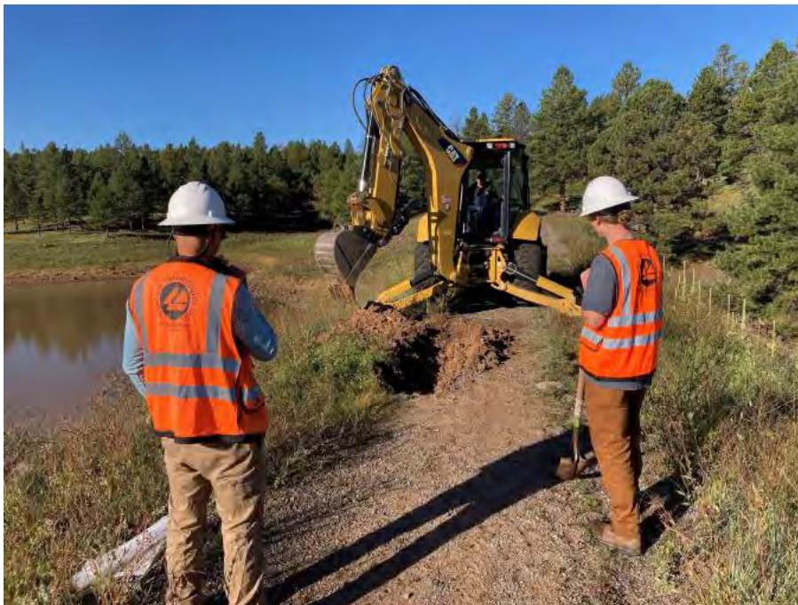
Upper Lake Mary Dam excavation.
