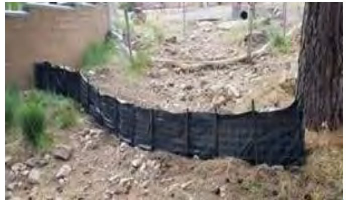
Properly installed silt fence prevents stockpiled sediment from migrating.
