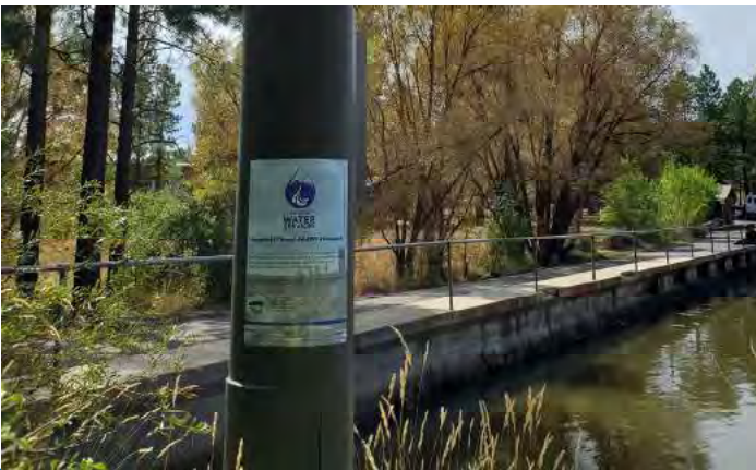
Flood Alert Gauge at the south end of Francis Short Pond.
