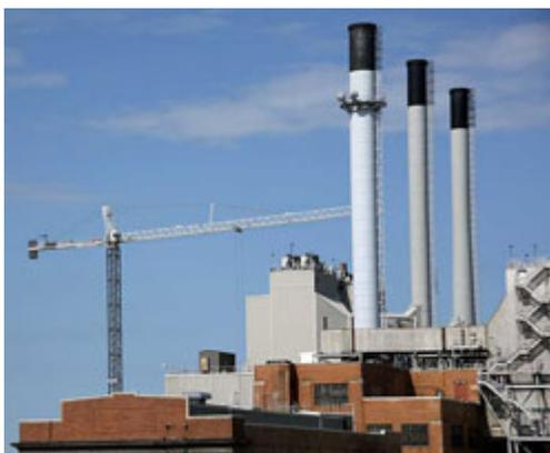
The stack has been reduced to 60 feet tall which is below the roof line of the surrounding buildings. The crews are continuing to demolish the stack walls, which get larger in diameter and wall thickness as the stack nears the ground.
