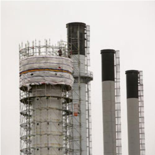
We're starting to see progress on the removal of the Blount stack. Crews have been hard at work removing the top of the stack. As pieces are removed, the plastic enclosure is moved down to continue to contain the dust and debris. This process is expected to last through October.
