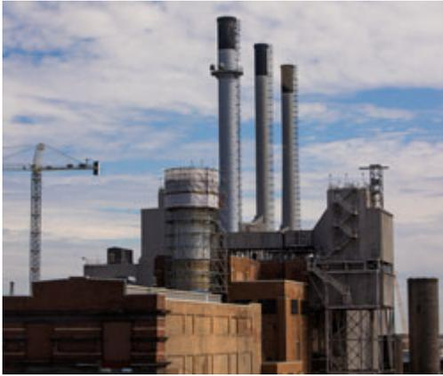
The crews have made substantial progress. The height of the stack, which was originally 244 feet, is expected to be under 100 feet by the end of the week. The wall thickens as it gets closer to the ground so the deconstruction may appear to slow down in the coming weeks. Since the project has started, crews have removed over 23 dumpsters of material contained in heavy-duty plastic enclosures.
