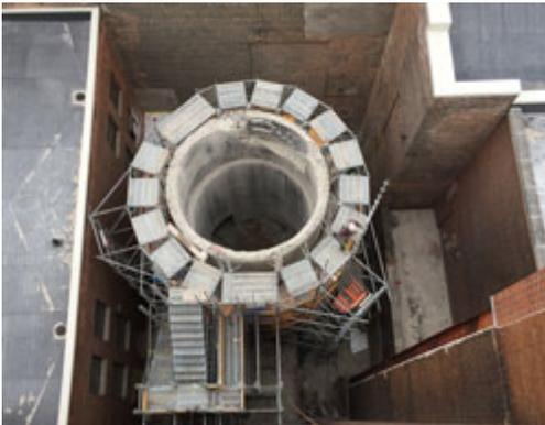
Since they started deconstructing the stack in July, contractor crews have removed more than 200 feet. Only about 40 feet of the stack remain, which is below the roof line of the surrounding buildings. Safety remains a focus as crews continue to demolish the stack walls.
