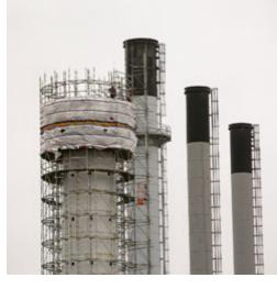
We're starting to see progress on the removal of the Blount stack. Crews have been hard at work removing the top of the stack. As pieces are removed, the plastic enclosure is moved down to continue to contain the dust and debris. This process is expected to last through October.
