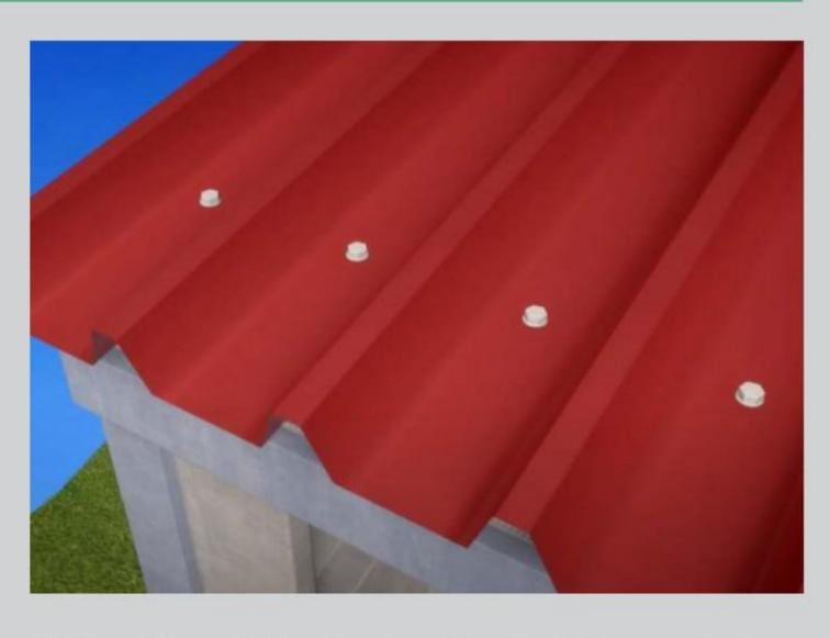
02. Place the metal sheet on top of the insulation sheet and fix with metal screws
