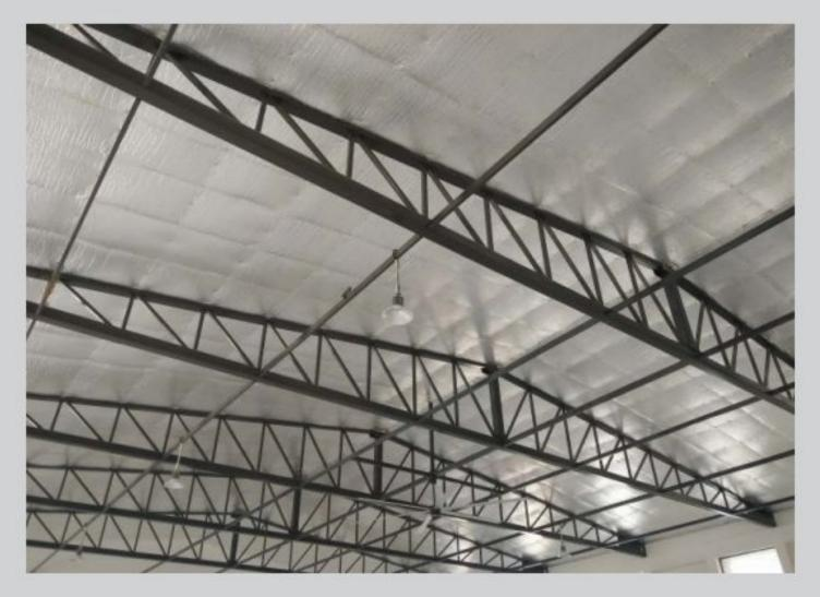
Under deck for existing building. (Retrofitting) When considering the applications for existing buildings, Aerolam products offer variety & best range to choose from. Aerolam insulation can be installed without removing the roofing sheet.
