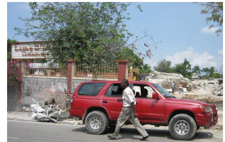
The administrative building can be seen on the left. On the right, the rubble left by the demolished building.
