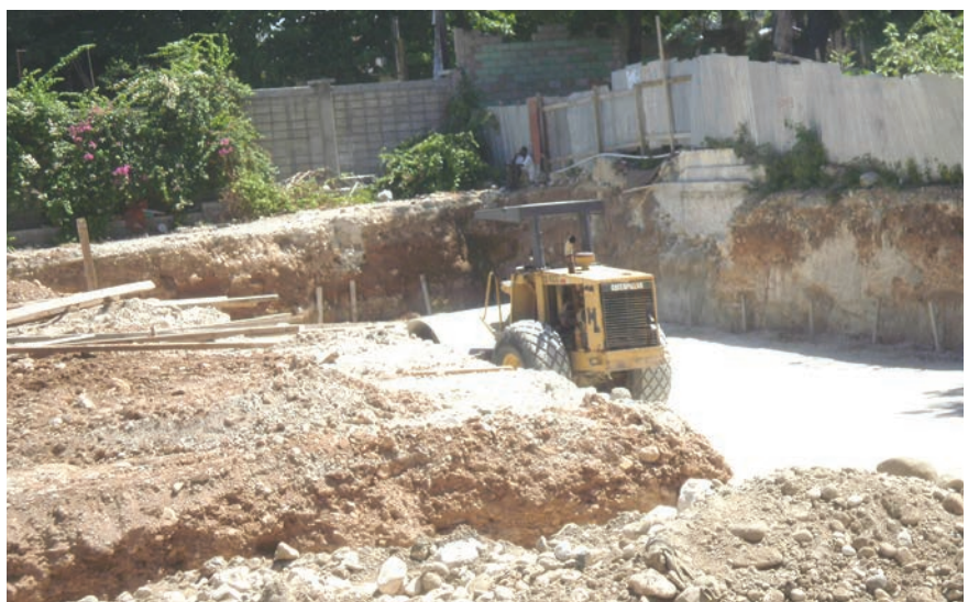
The reconstruction has started at the Canado Haitian Secondary School.
