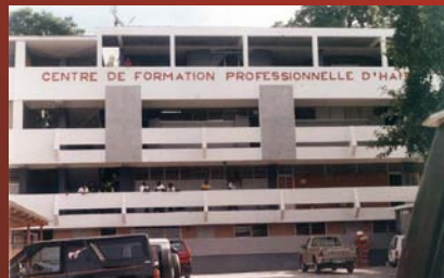
CANADO TECHNICAL SCHOOL PORT-AU-PRINCE
