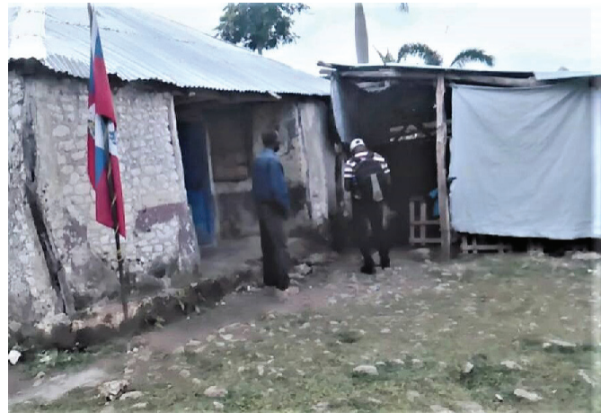
Laguamite School: School's exterior view.
