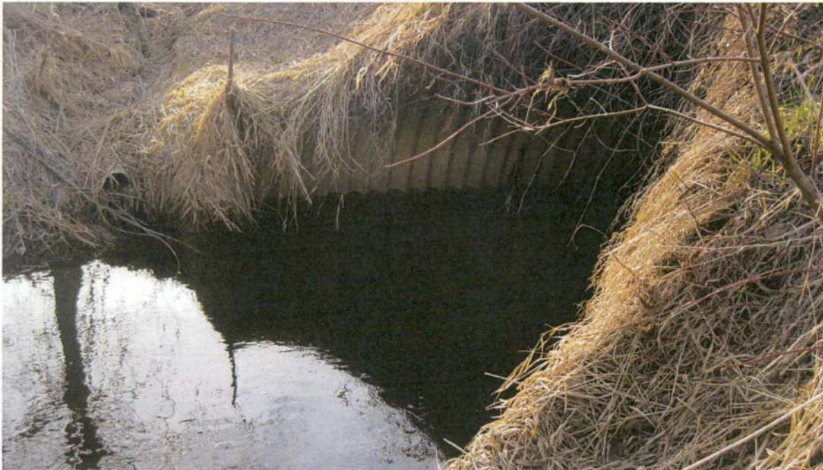
Picture No. 10 shows the northern upstream end of the 8.5-foot by 13-foot arch CSP culvert crossing 108 th Street.
