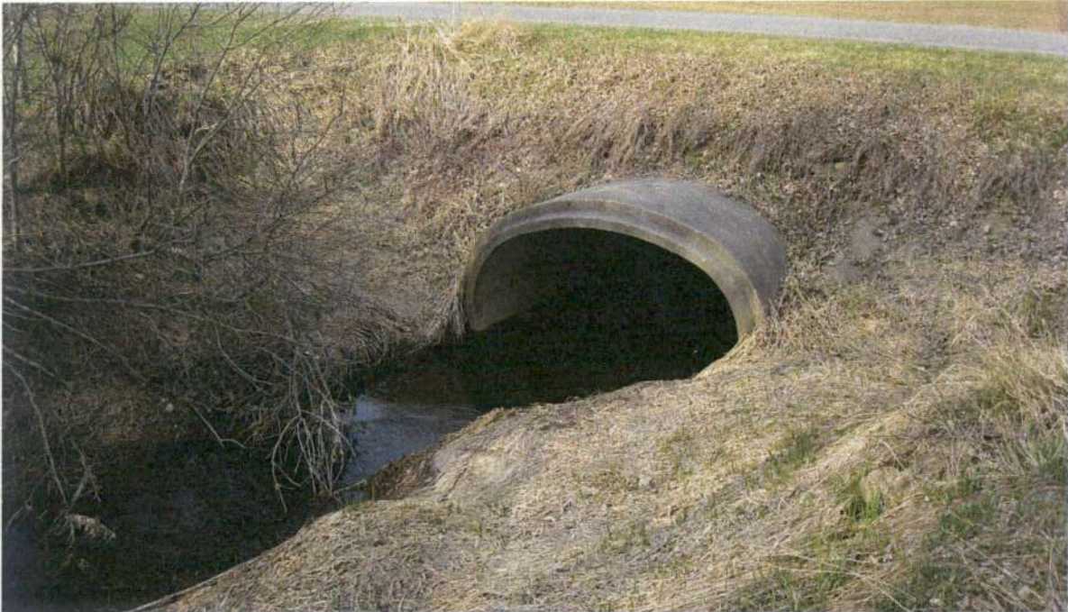
Picture No. 15 shows the downstream eastern end of the 5-foot by 9-foot elliptical RCP culvert crossing under East Paris Ave. Picture is taken looking southwest.
