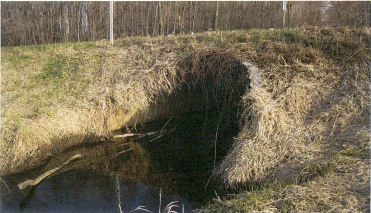
Picture No. 9 shows the southern downstream end of the 8.5-foot by 13-foot arch CSP culvert crossing under 108 th Street. Picture is taken looking northwesterly.
