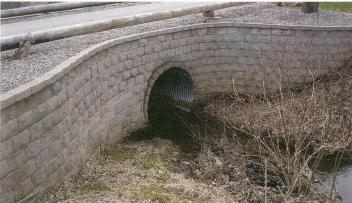
Picture No. 18 shows the western upstream end of the 66-inch CSP culvert. Picture is taken looking southeast.
