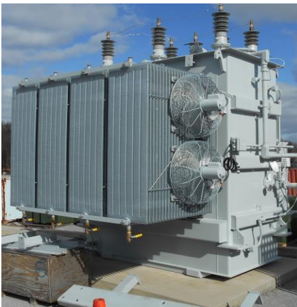
34.5 kV TRANSFORMER INSTALLATION, MD
