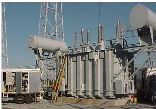
230 kV AUTOTRANSFORMER INSTALLATION, MD
