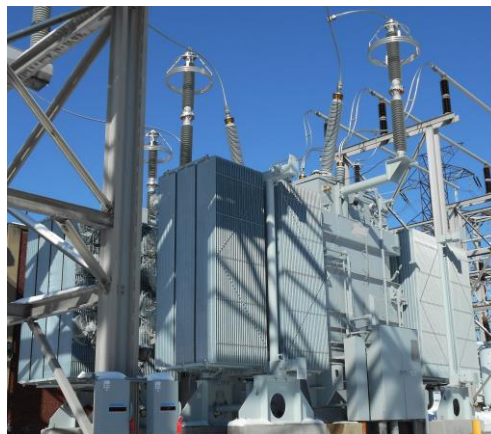
345 kV AUTOTRANSFORMER REFURBISH AND COOLING UPGRADE, PA
