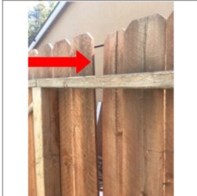
•Sections of wooden fencing showed signs of moisture damage and possible insect damage. Recommend repair damaged sections as needed.
