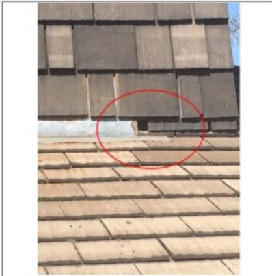
•Flashing had Pulled away from chimney. Recommend repair. •Some sections of flashing at eaves edge was damaged/missing. Recommend repair.
