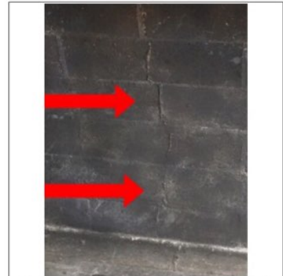
•Open joints or cracks in firebrick of fireplace. Recommend properly sealing and repair.
