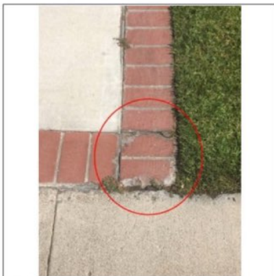
•Driveway had some settlement cracks and damaged bricks. Recommend repair.
