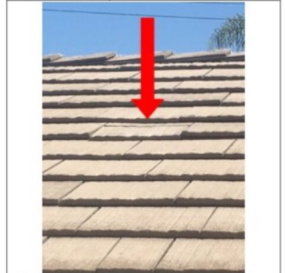
•Roof had damaged and missing concrete tile shingles. Recommend licensed roofing contractor inspect and evaluate further for repairs.
