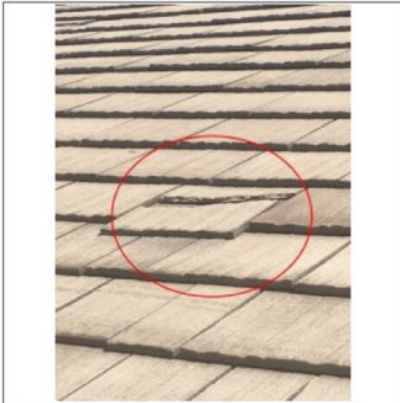
•Roof had damaged and missing concrete tile shingles. Recommend licensed roofing contractor inspect and evaluate further for repairs.
