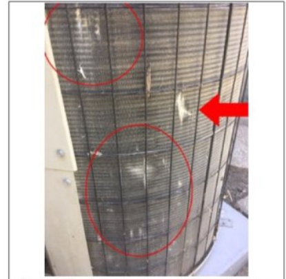
•Outside condenser unit coils on AC unit were damaged. Recommend licensed HVAC technician inspect and evaluate further for repairs.
