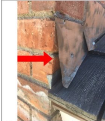
•Flashing had Pulled away from chimney. Recommend repair. •Some sections of flashing at eaves edge was damaged/missing. Recommend repair.
