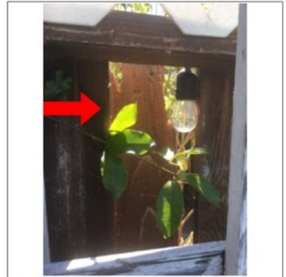
•Sections of wooden fencing showed signs of moisture damage and possible insect damage. Recommend repair damaged sections as needed.
