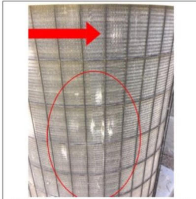
•Outside condenser unit coils on AC unit were damaged. Recommend licensed HVAC technician inspect and evaluate further for repairs.
