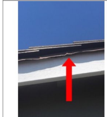
•Flashing had Pulled away from chimney. Recommend repair. •Some sections of flashing at eaves edge was damaged/missing. Recommend repair.
