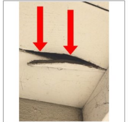
Soffit damaged/rotted, recommend repair by licensed contractor.
