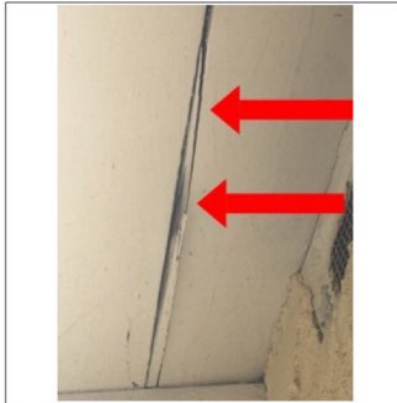
Soffit damaged/rotted, recommend repair by licensed contractor.
