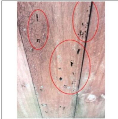
Backyard wooden fence had some damaged/rotted wooden planks. Recommend repair or replace as needed. Evidence of termite damage found in some of the wooden planks. Recommend licensed termite contractor inspect and evaluate further for repairs.
