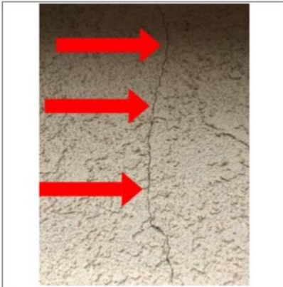
Siding had some damage/cracking recommend repair by licensed contractor.
