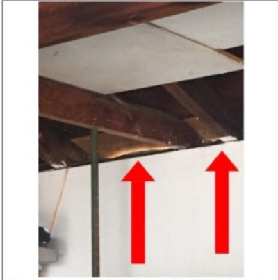
Recommend licensed contractor inspect and evaluate interior garage walls to repair visible gaps to exterior of garage wall.
