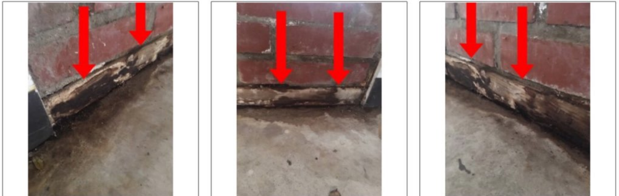
Sill plates in garage were rotted/water damaged recommend repair/replacement by qualified licensed contractor.
