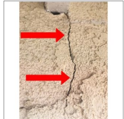
Siding had some damage/cracking recommend repair by licensed contractor.
