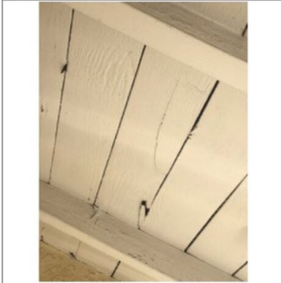
Soffit damaged/rotted, recommend repair by licensed contractor.
