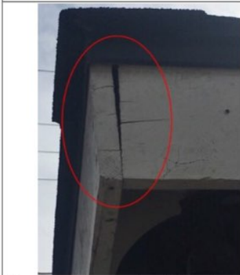
Garage Trim and soffit had some damage recommend repair by licensed contractor.
