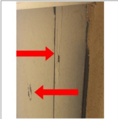
Soffit damaged/rotted, recommend repair by licensed contractor.
