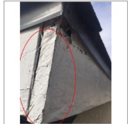
Garage Trim and soffit had some damage recommend repair by licensed contractor.
