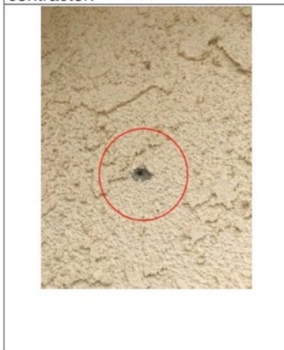
Cracks/holes in stucco siding recommend repair by licensed contractor.
