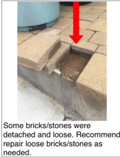
Some bricks/stones were detached and loose. Recommend repair loose bricks/stones as needed.
