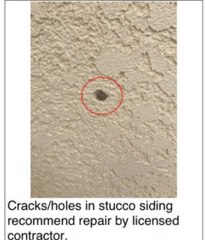
Cracks/holes in stucco siding recommend repair by licensed contractor.
