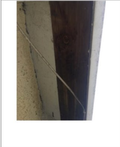
Soffit damaged/rotted, recommend repair by licensed contractor.
