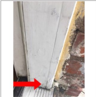
Entry door weathered, recommend paint/stain to protect from further damage.
