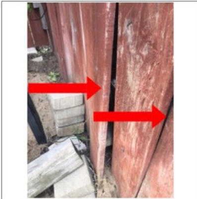
Backyard wooden fence had some damaged/rotted wooden planks. Recommend repair or replace as needed.
