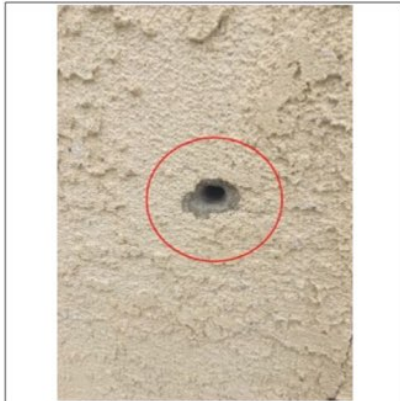
Cracks/holes in stucco siding recommend repair by licensed contractor.
