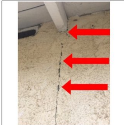
Cracks/holes in stucco siding recommend repair by licensed contractor.
