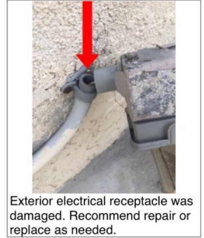
Exterior electrical receptacle was damaged. Recommend repair or replace as needed.
