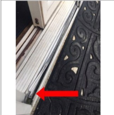
Patio door does not slide easily, rollers damaged. Recommend repair/replace as needed.
