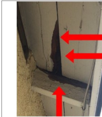
Soffit damaged/rotted, recommend repair by licensed contractor.
