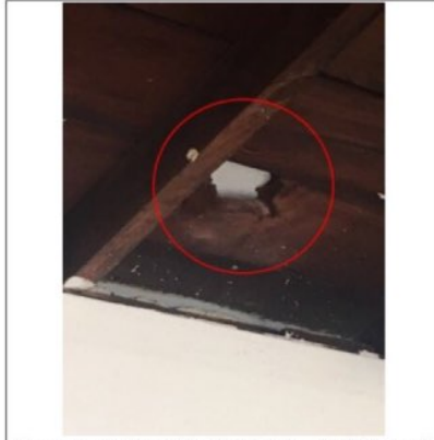
Damaged roof planks in ceiling of garage roof. Recommend licensed contractor inspect and evaluate further for repairs.
