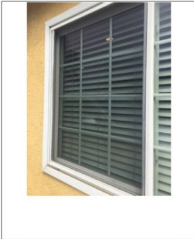
Trim around window was in need of maintenance, sanding, repainting.
