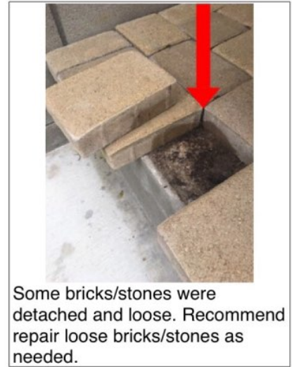
Some bricks/stones were detached and loose. Recommend repair loose bricks/stones as needed.
