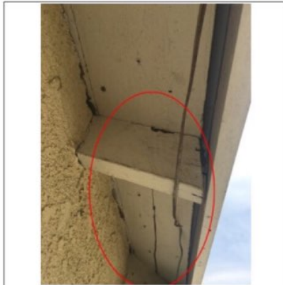
Garage Trim and soffit had some damage recommend repair by licensed contractor.
