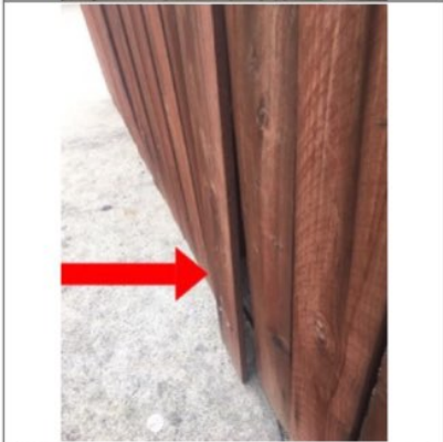
Driveway gate was damaged and bent. Does not close easily. Recommend repair or replace as needed.
