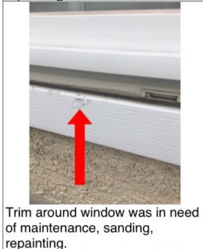
Trim around window was in need of maintenance, sanding, repainting.
