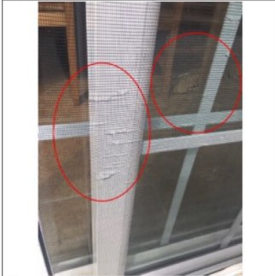
Screen patio door was damaged and torn. Recommend replace.
