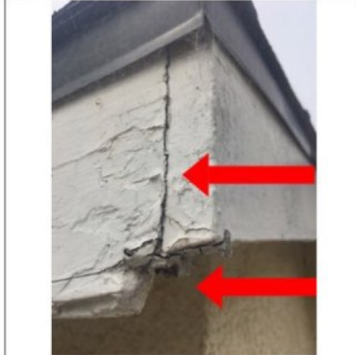
Trim had some deterioration recommend repair and painting. Some loose and missing trim recommend repair. Some rotted/damaged trim boards recommend repair/replacing damaged sections. Recommend repair of damaged trim by a qualified licensed contractor.
