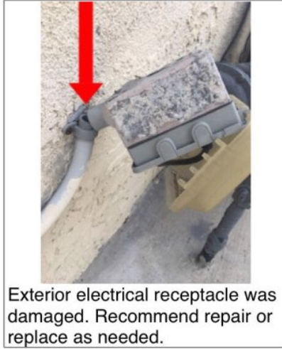
Exterior electrical receptacle was damaged. Recommend repair or replace as needed.
