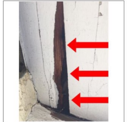
Soffit damaged/rotted, recommend repair by licensed contractor.
