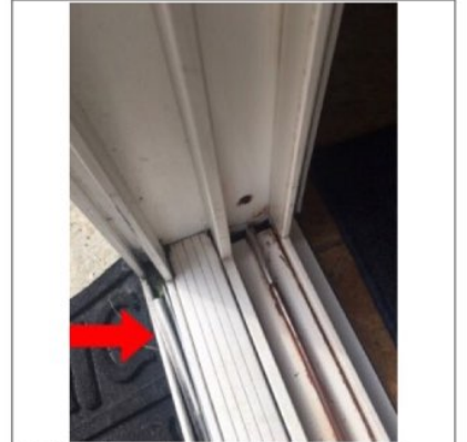
Patio door does not slide easily, rollers damaged. Recommend repair/replace as needed.
