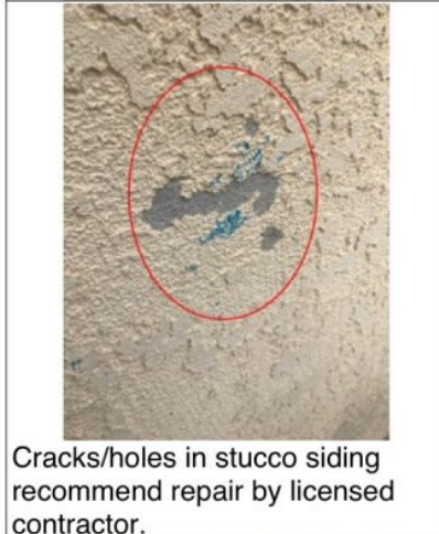
Cracks/holes in stucco siding recommend repair by licensed contractor.
