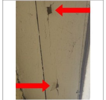
Soffit damaged/rotted, recommend repair by licensed contractor.
