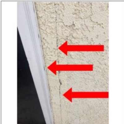
Siding had some damage/cracking recommend repair by licensed contractor. Garage Trim/soffit had some damage recommend repair by licensed contractor.
