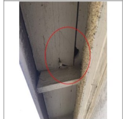
Garage Trim and soffit had some damage recommend repair by licensed contractor.
