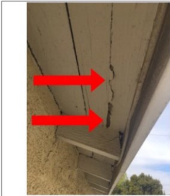
Soffit damaged/rotted, recommend repair by licensed contractor.
