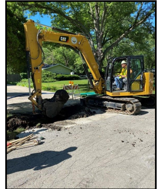
BURR OAK ROAD STORM DRAIN PROJECT
