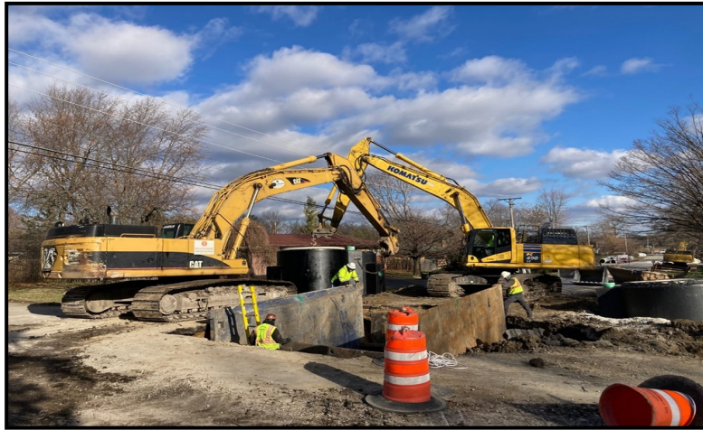
Wheaton Sanitary District - Northside Interceptor—Sewer Replacement Armbrust Ave. & Ellis Ave.
