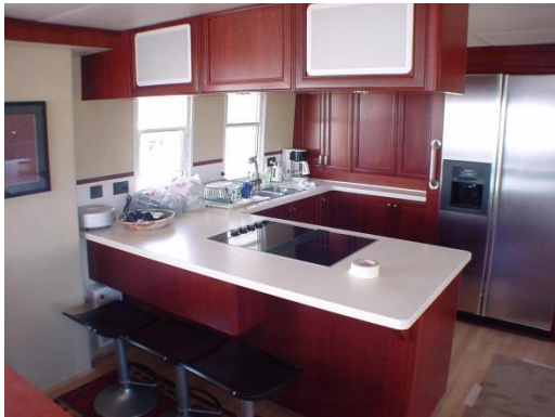
Dropped valance in wood – allows room for wire raceways and light fixtures
