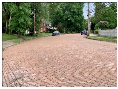
View of Graham Boulevard near Laketon Road has a brick surface nearly a hundred years old. Much of the surface is just as flat and secure in 2023 as it was when it was laid in the 1920s.
