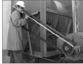
Using a straight edge to check alignment
