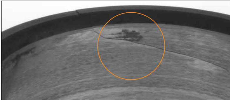
Fig. 51. This ball bearing inner ring fracture is a result of being installed on top of a metal contaminant or raised metal nick.
