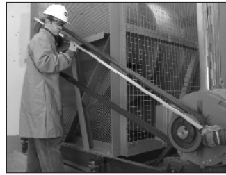
Using a straight edge to check alignment
